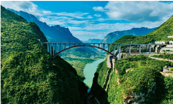
Wumengshan Bridge on the Nayong-Qinglong Expressway
